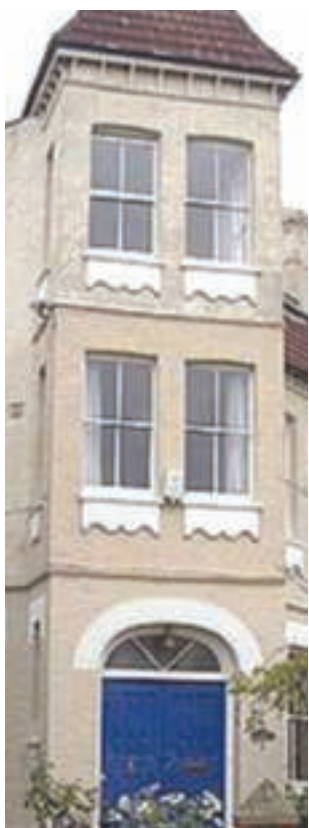
The Foster's home in Bromley, Kent
